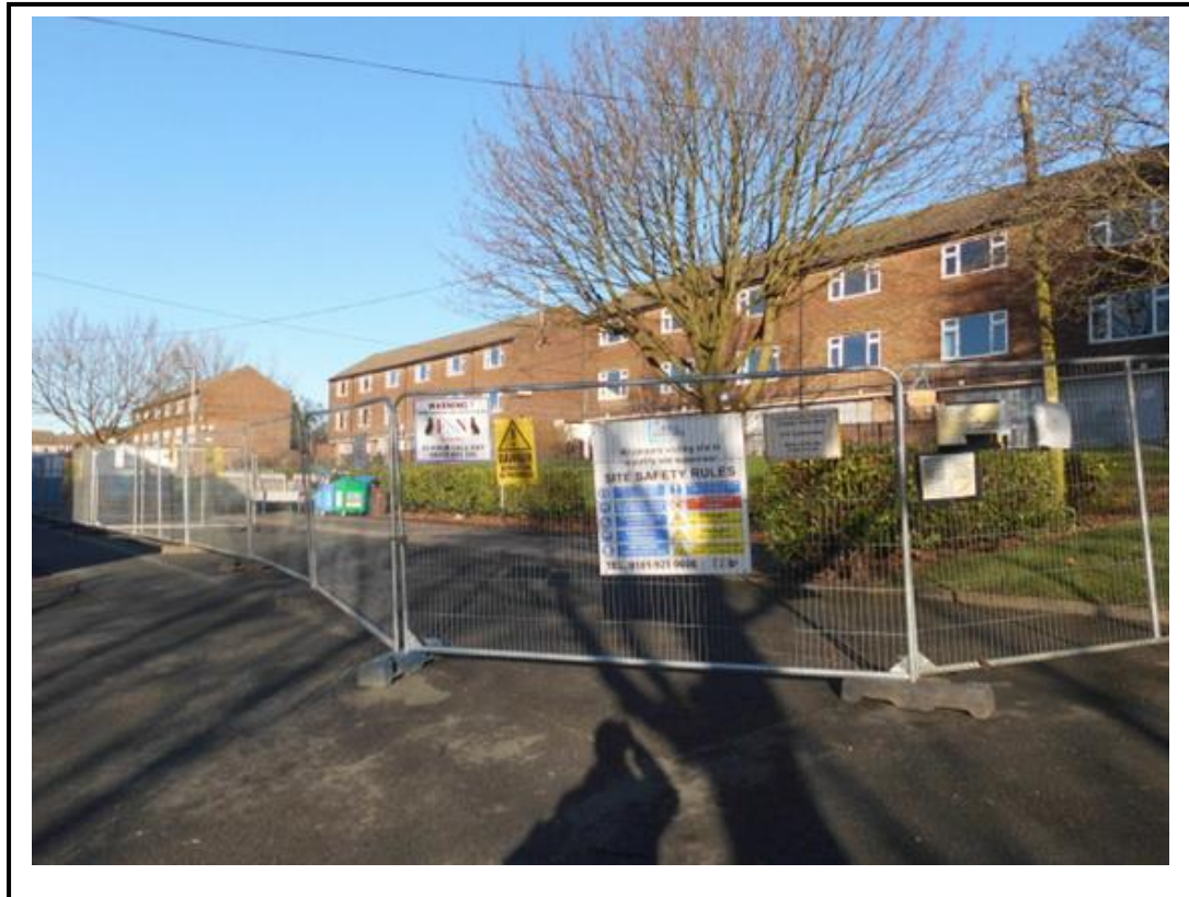
Photo 3 Rydal Walk Maisonettes prior to demolition
